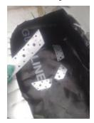
Screw down perforated hoop iron around downpipe edge. Don't overtighten the screws. You will need 200mm of hoop iron for a 200mm round down pipe. For square downpipes, cut to measure each side and overlap at corners.
