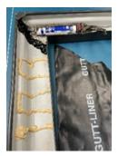
Apply adhesive in castle pattern to within 200mm of corner and apply black silicone to the join in the gutter as shown.
