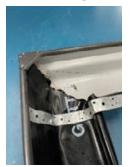
Place one end of hoop iron under outer lip of gutter to secure. Mould to fit existing profile and secure with screw on upper side wall under roof overhang. Installing hoop iron to corners will hold GUTTA-LINER down flat onto black silicone ensuring it is water tight.
