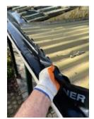
Lay liner onto adhesive within gutter and smooth out flat. Push liner up under the exposed outer, turn back lip of gutter so no water will get behind liner.
