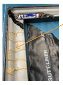
Apply a continuous bead of adhesive along the gutter in a 'castle' pattern (100–150mm apart).
