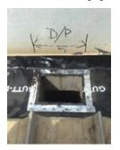
Find the middle of the downpipe. Cutting from the middle to the edge first, cut out the GUTTA-LINER so the whole downpipe is open ensuring there is no restriction to the outlet.
